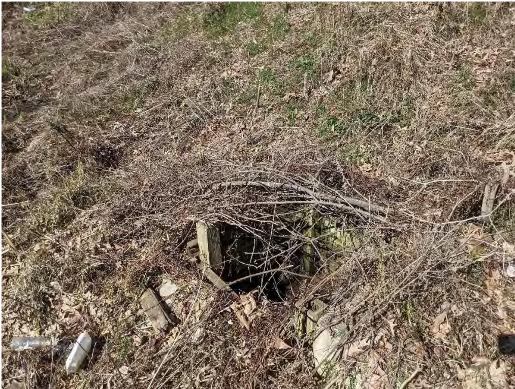
Photo 20: View of SW-M17 (OCS1982) located south of Lot P13.
