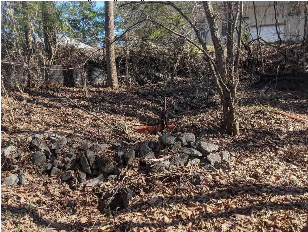
Photo 12: View of SW-M10 (for sheet flow) off the northeast corner of the Student Competition Team Building.
