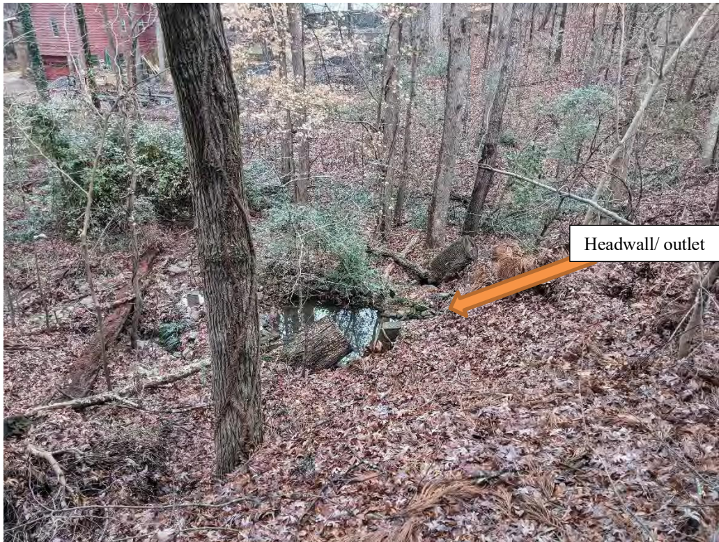
Photo 6: View of SW-K06 located north of the North Parking Deck.
