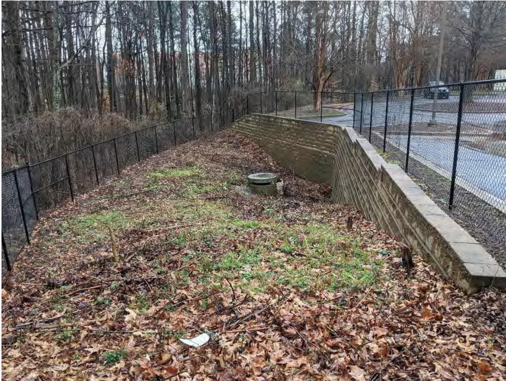
Photo 17: View of outfall SW-M14 (OCS15) located east of the Gymnasium.
