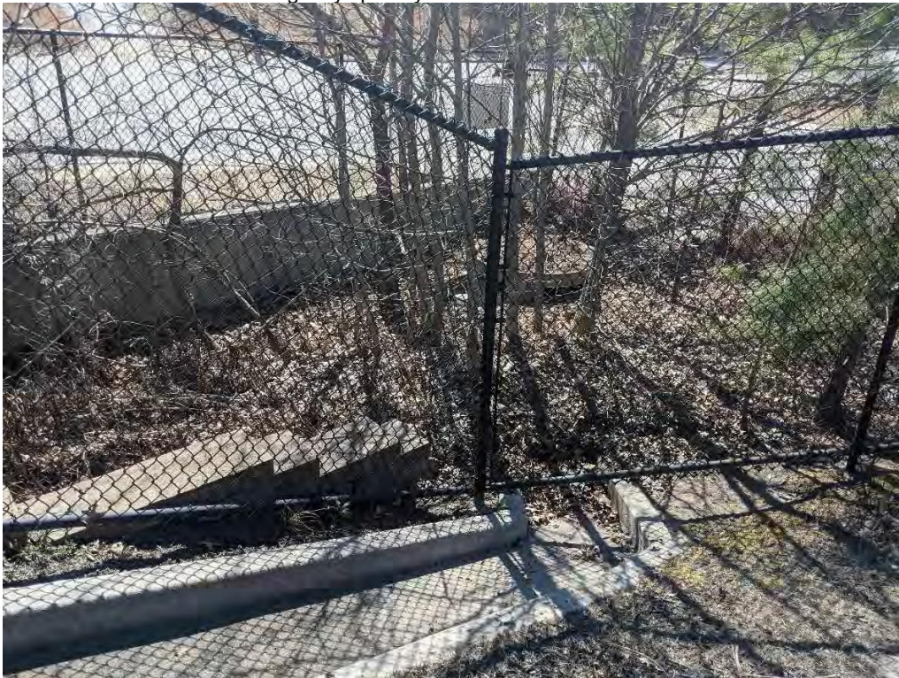
Photo 20: View of wier inlet located in the south side of the Perch entrance drive. Discharges to SW-K13.
