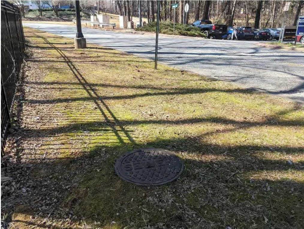
Photo 19: View of SW-M16 (JB-19) located south of University Commons.
