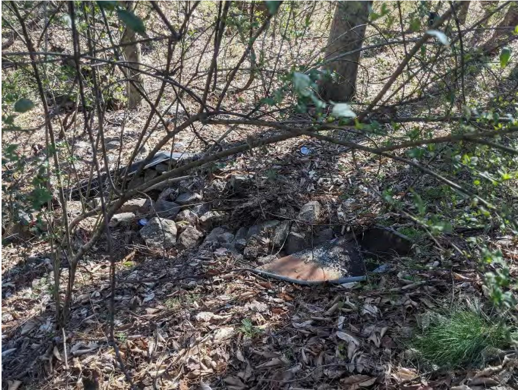
Photo 7: View of SW-M06 located along Alumni Drive, south of the softball fields and Lot P40.
