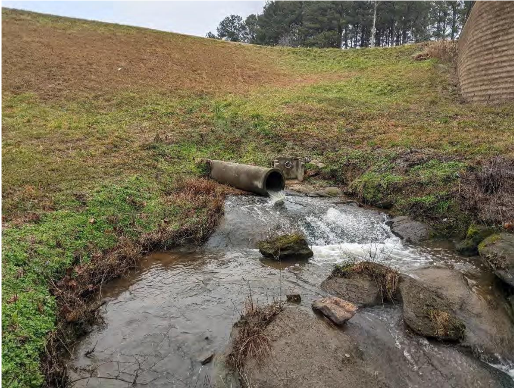
Photo 17: View discharge from outlet control structure within Nelson Pond, located on south side of the Category1 dam.
