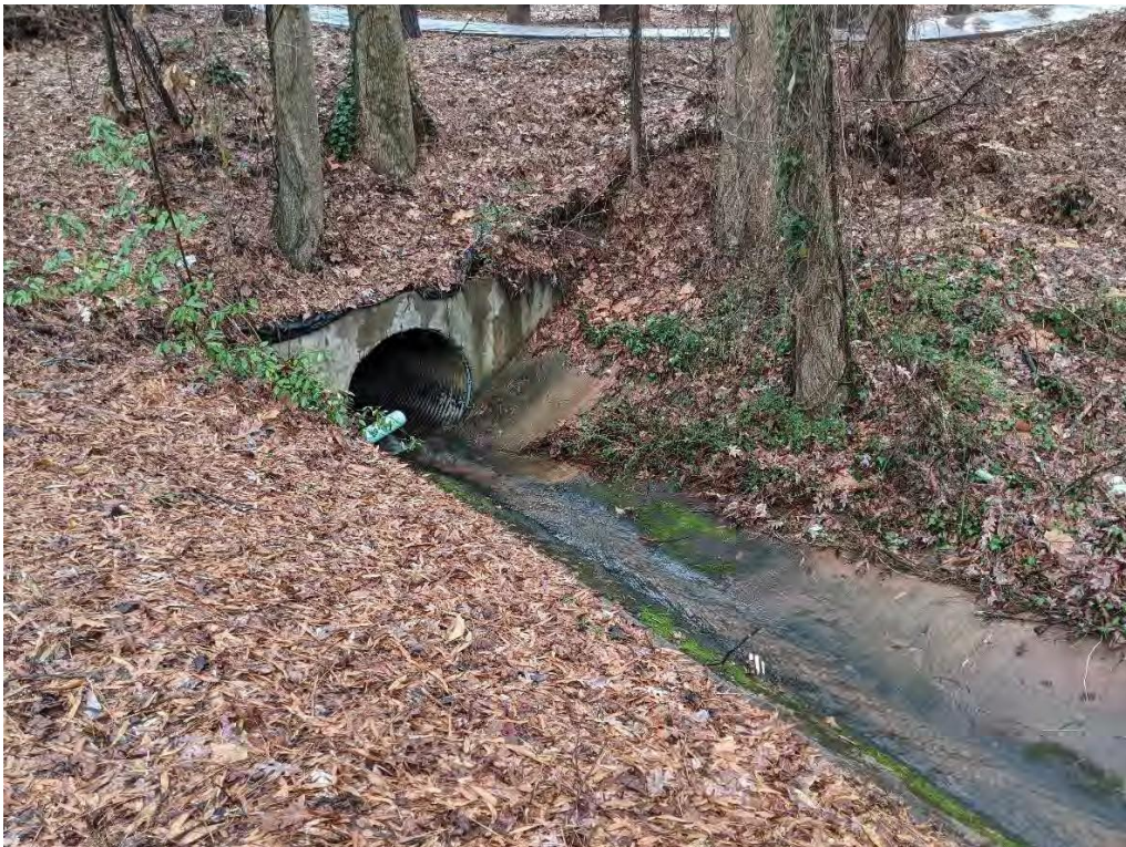
Photo 18: View of outfall SW-M15 (the end of the concrete channel) located on the west side of University Commons.
