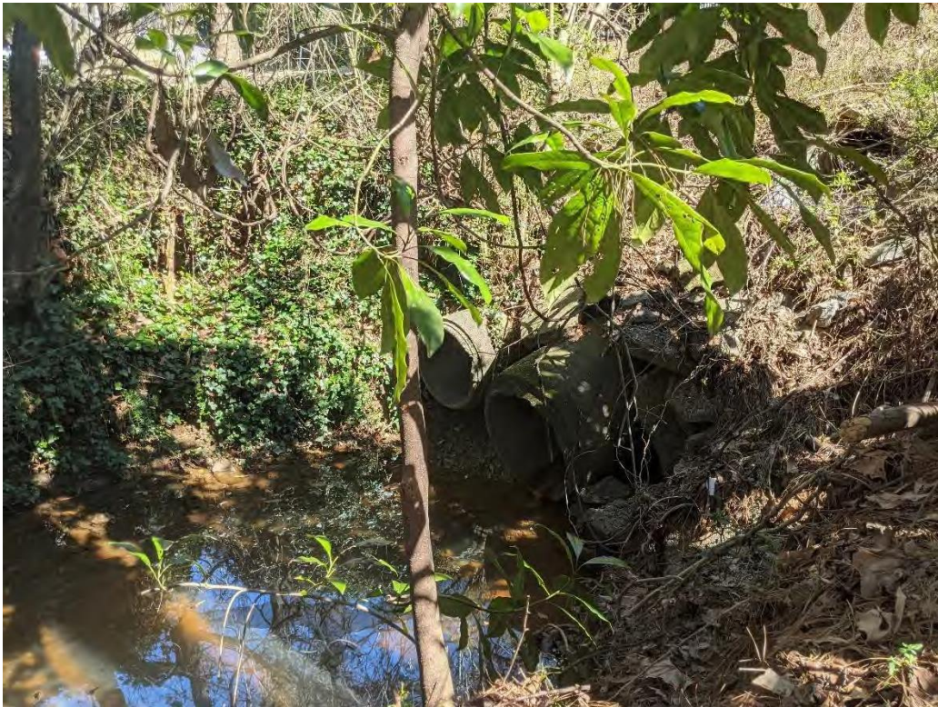
Photo 4: View of SW-K04, located west of the Social Sciences building.
