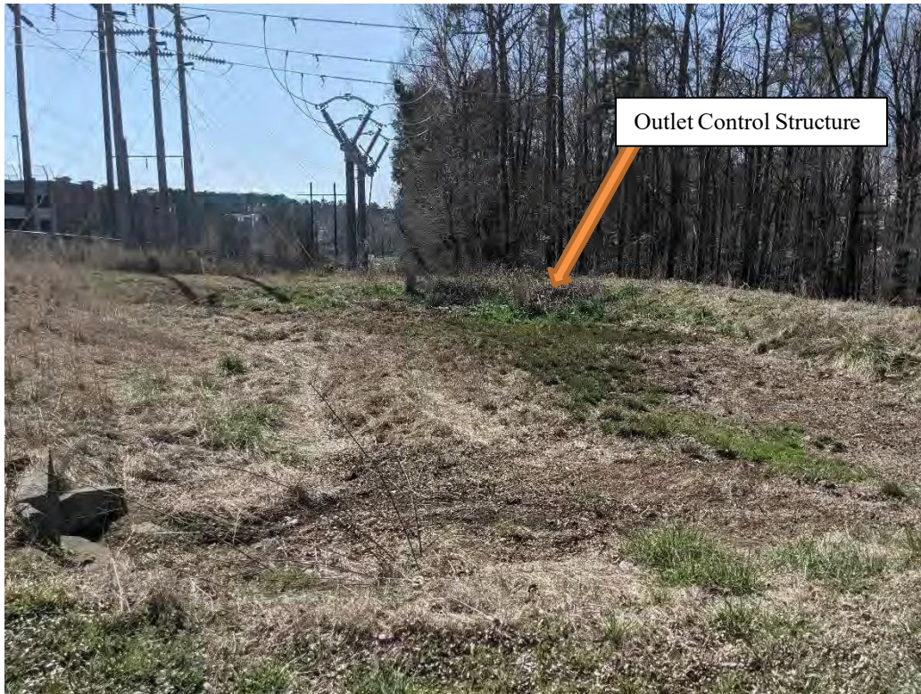
Photo 25: View of detention pond and outlet control structure (OCS8053) discharging to SW-M21 located near Facilities building.
