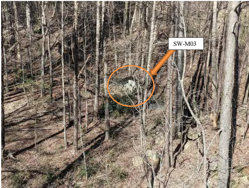
Photo 3: View of SW-M03 (headwall) located southwest of West Parking Deck P60.
