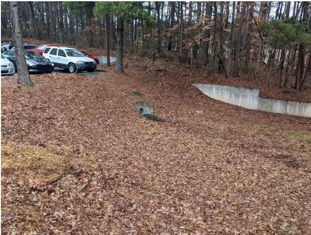
Photo 8: View of headwall (HW05) and detention area discharging to outfall SW-K07.
