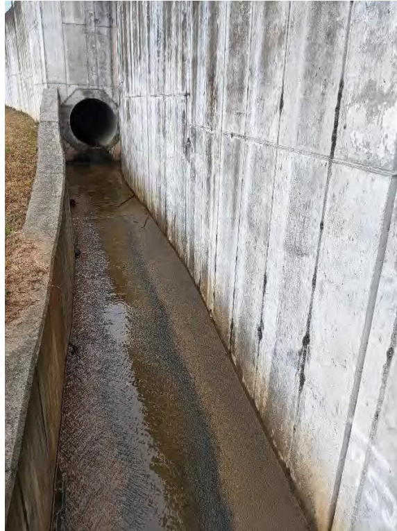
Photo 19: View of concrete pipe discharging into concrete channel located on southern portion of Nelson Pond emergency spillway.
