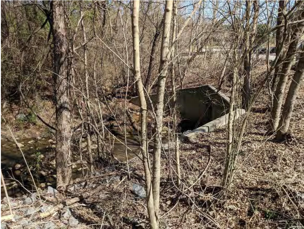
Photo 21: View of SW-K13, along Big Shanty Road, which serves as the main discharge point for stadium area.
