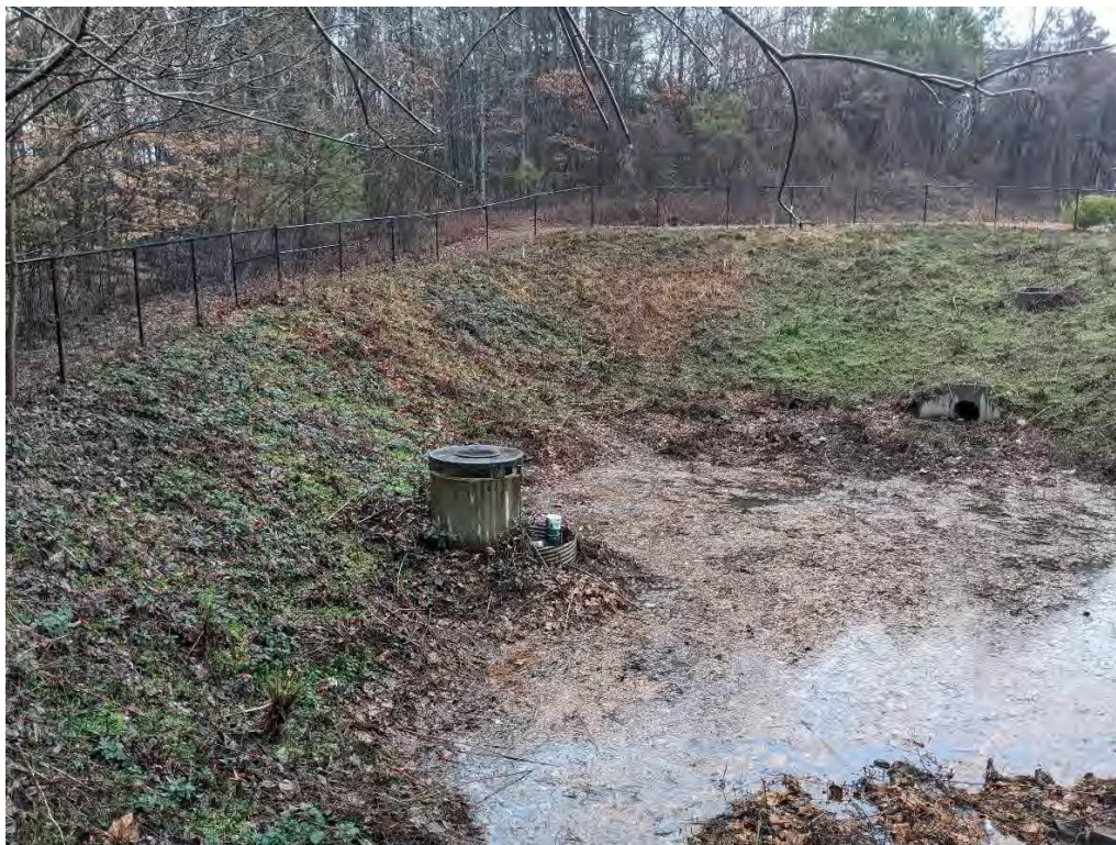
Photo 4: View of pond and outlet control structure (OCS2941) directly upstream of SW-M03.
