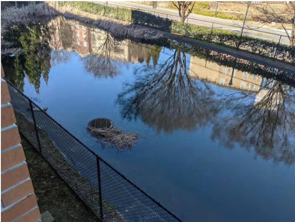
Photo 10: View of outfall SW-K08 located within pond near Central Deck.
